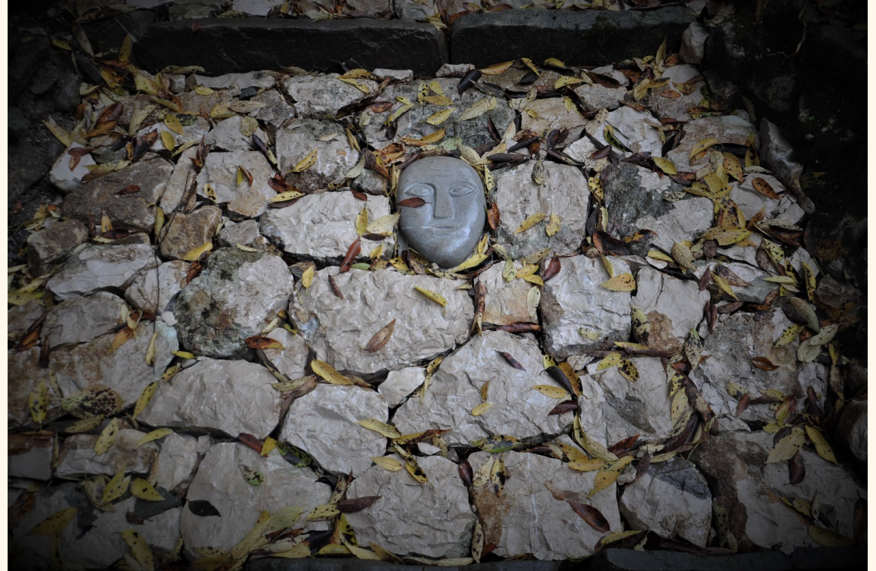
Detail of the kalderimi (cobblestone pathway) constructed during the apprenticeship. Photo by Grigoris Koutropoulos
